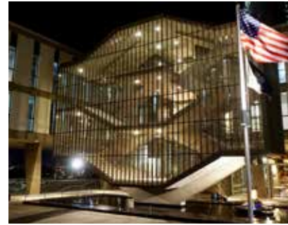
Staircase Renovation: Work is finished on the glass-enclosed staircase affectionately known as the "birdcage" with $1,015,000 in county funds.
